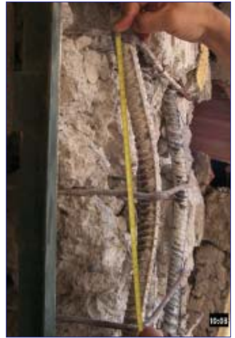
Figure 5: Non adequate detailing
