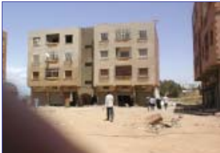
Figure 2: Soft (first) storey
