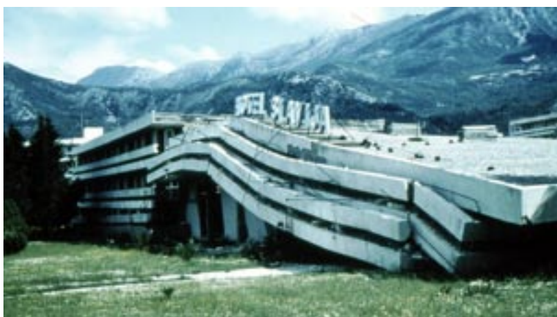
Fig.2. Left picture: destroyed building during the 1963 destructive earthquake of Skopje, Macedonia (magnitude 6.2). Right picture: collapsed hotel structure in Montenegro during the 1979 earthquake (magnitude 7.0).
