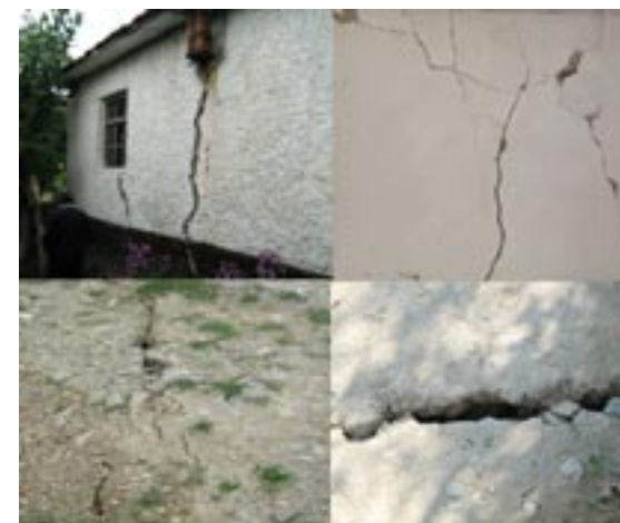
Figure 3 - Views of ruined buildings in Qerenecy village and ground cracks (Zaçaj, M et al. 2009, Field Report)
