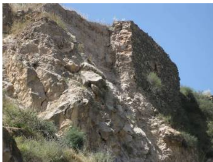
Figure 4.2.1f: Close up of the fall of part of an old retaining wall. It can be observed that the intrados filling remains meta-stable. This type of instability also appears on the south face of Lorca's castle cliff (see figure 2.1).
